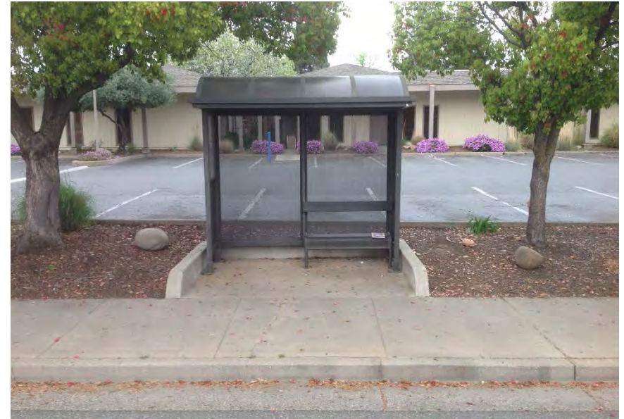
FIGURE 4-31. TRANSIT SHELTER AT THE MEDICAL CENTER TRANSIT STOP
